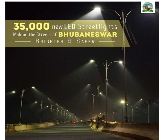
LED Lighting in Bhubaneswar Smart City India
